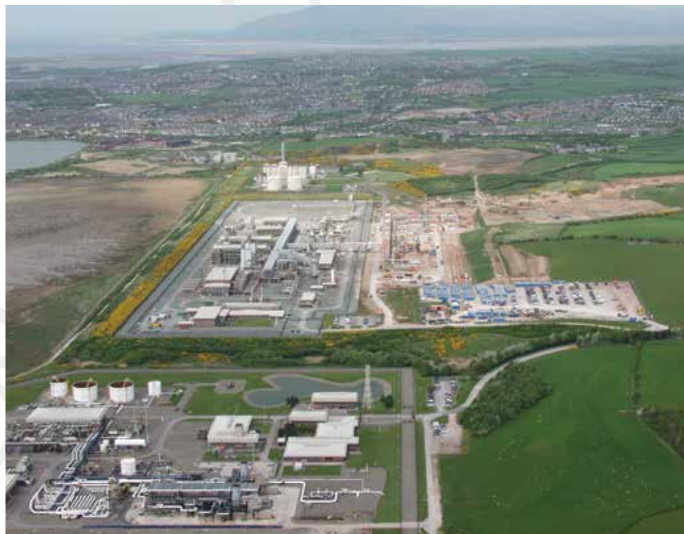
Commissioned in 1994 , Spirit Energy Ltd.'s North Morecambe onshore terminal at Barrow-in-Furness, Cumbria, UK, uses a unique process configuration combined with adsorbents from BASF Corp. to achieve gas specifications for cryogenic processing and transportation into the UK's national grid. Photo from Costain Group PLC.
