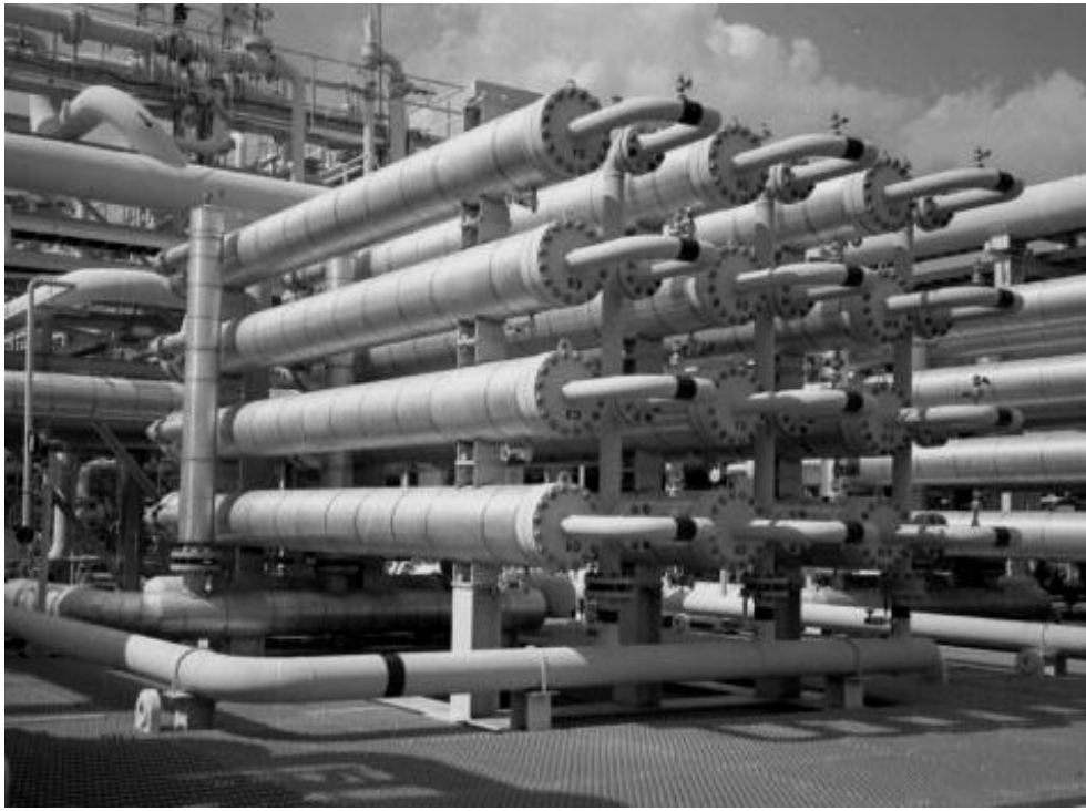
Figure 9. Skid Containing Air Liquide Membrane Elements
