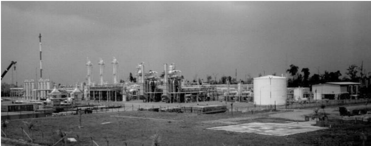
Figure 1. Grissik Gas Plant
